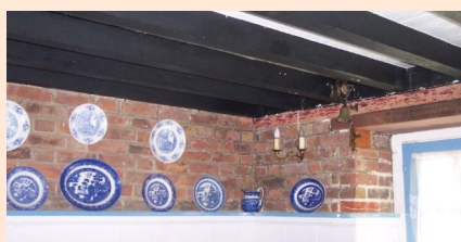
Exposed beams, unfaced brick and wooden dado panelling.
