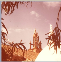
Bell Tower repairs 1974
